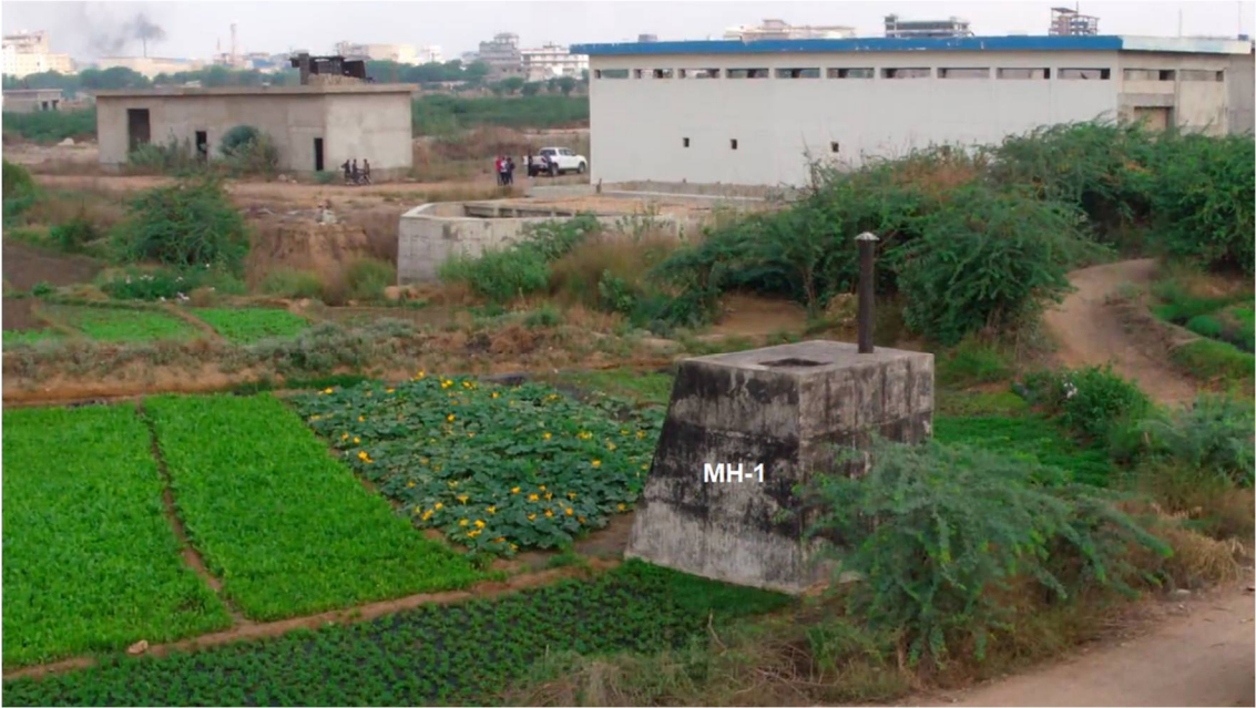
Figure 9. Location of Manhole MH-1 on Raw Wastewater Interceptor
